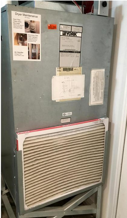
*Figure 1 - Fan Coil Unit*
