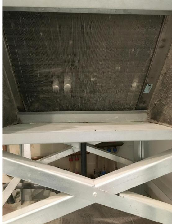
*Figure 2 - Fan Coil Radiator*
