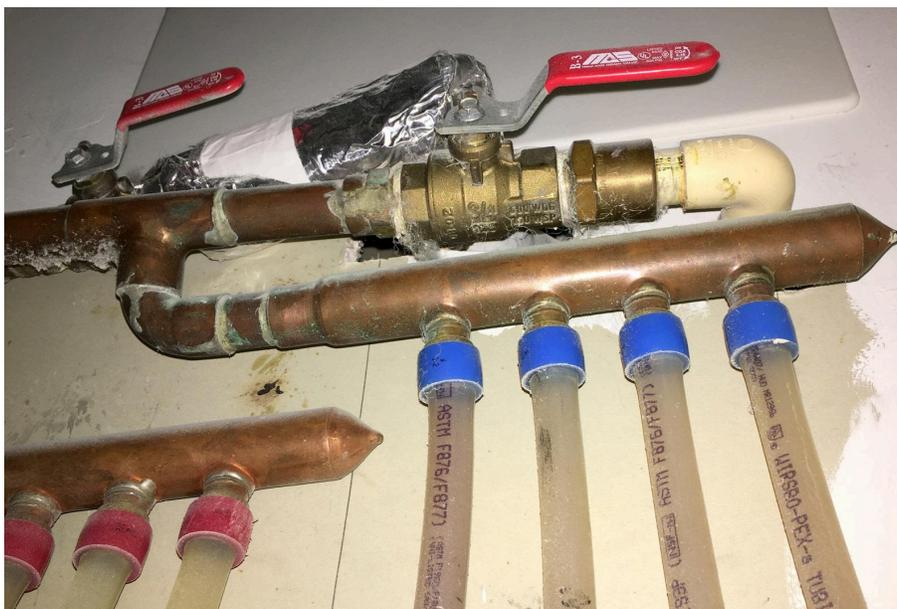
*Figure 8 - Hot and Cold Water Shut OFF Valves*
