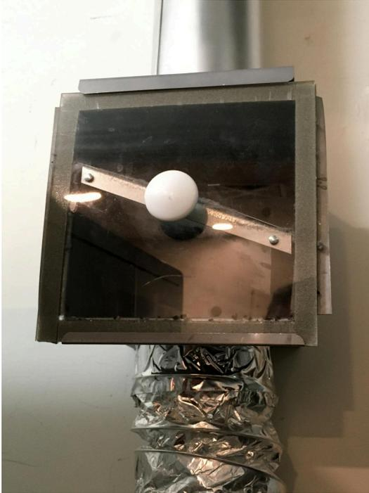
Figure 5 - Metal Box with Lint Filter
